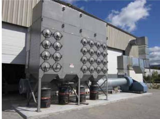
The cartridge dust collection system was designed so that incoming dust and solid materials pulled from machines like the router above first enter an empty plenum. This enables turning “bird nests” and other heavier pieces to fall to the bottom of that plenum without damaging any cartridges. The airstream with dust then enters cartridge-filled plenums on either side of the empty one, and clean air is returned to the facility.
